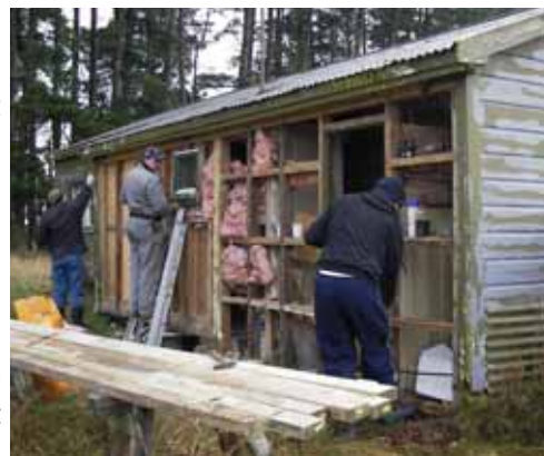
Lodge Custodian Linz Withington supervising building works at Castle Rock.
